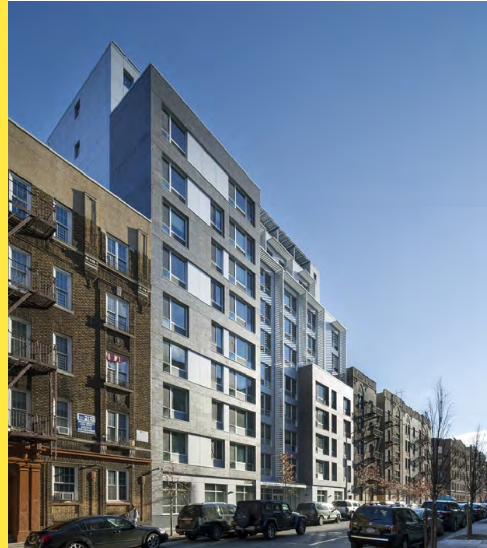
Completed, Creston Ave, Bronx, NY
