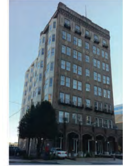
The Commons at Imperial Atlanta, GA 100 Units
