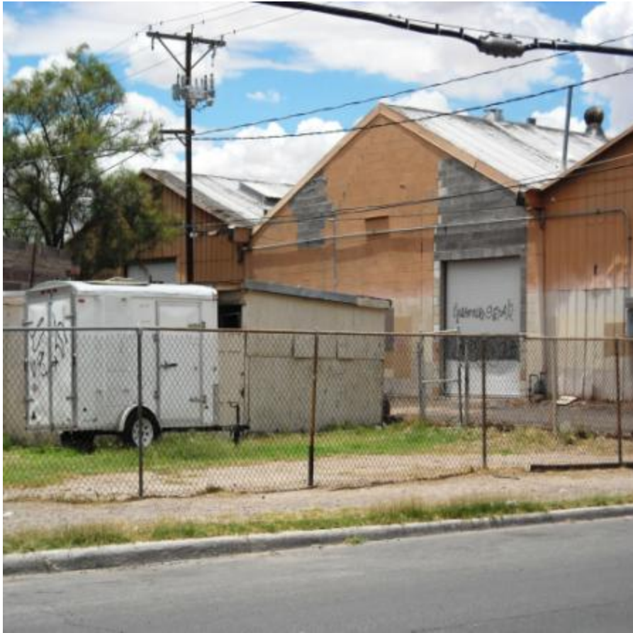
Lack of exterior maintenance and esthetics
